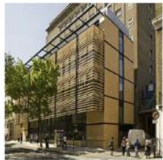
Engineering Front Building Staff: 21 12 mins
